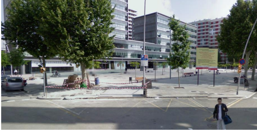
Figure 1.9: Picture of the selected smart parking test facility
